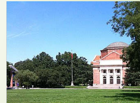
Built in 1917, the Grand Auditorium with its Jeffersonian architectural design is a centerpiece of the old campus
